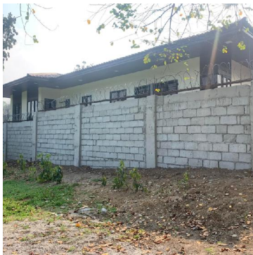
HOLE # 3 SOUTH COURSE PERIMETER FENCE
