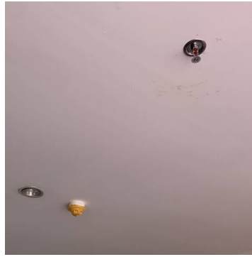
AUTOMATIC FIRE SPRINKLER & DETECTION ALARM
