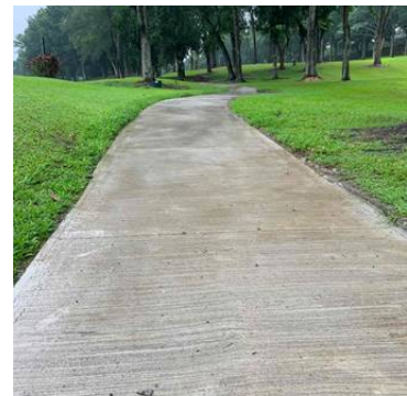
CART PATH REPAIR WORKS
