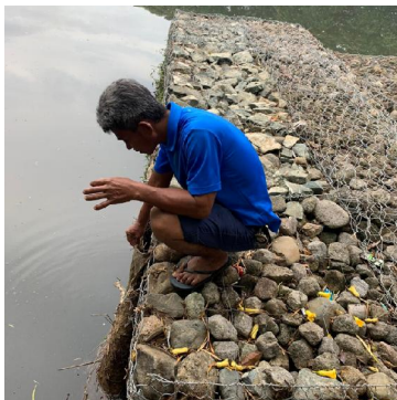
GABION FILTER MAINTENANCE WORKS
