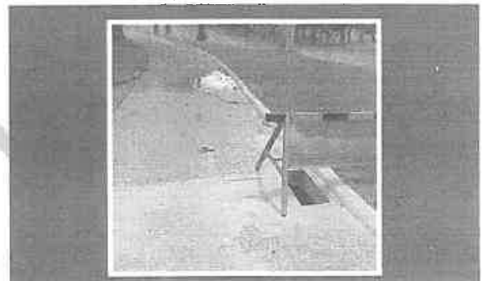
SOUTH COURSE HOLE #1 CONSTRUCTION OF GUTTER
