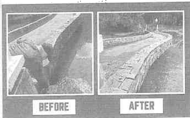
SOUTH COURSE BRIDGE #10 REPAIR OF GREEN SLATE
