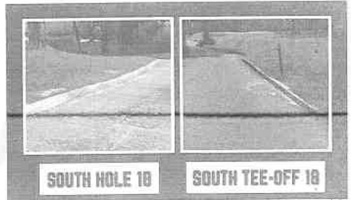
REPAIR OF CONCRETE GUTTERS
