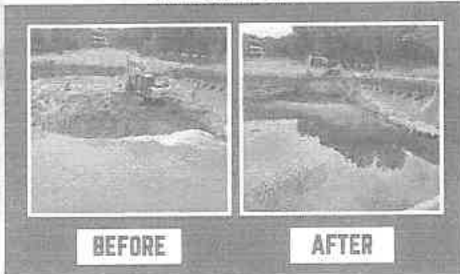
NORTH COURSE HOLE #9 DREGGING OF SILT
