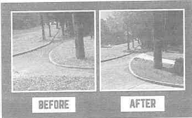
SOUTH COURSE HOLE #4 CONSTRUCTION OF CART PATH
