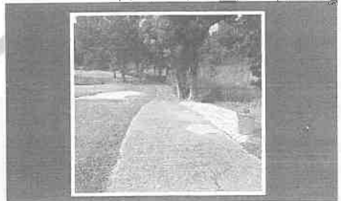
NORTH COURSE HOLE #12 CONSTRUCTION OF LAY-BY
