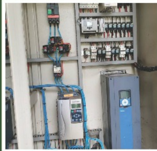
SOUTH COURSE PUMP HOUSE CONTROL PANEL INSTALLATION OF VARIABLE FREQUENCY DRIVES
