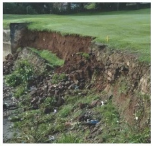
NORTH COURSE HOLE #9 REPAIR OF RIPRAP WALL SLOPE
