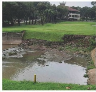
NORTH COURSE HOLE #9 REPAIR OF RIPRAP WALL SLOPE
