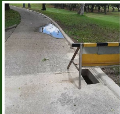
SOUTH COURSE HOLE #1 CONSTRUCTION OF GUTTER
