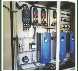
SOUTH COURSE PUMP HOUSE CONTROL PANEL INSTALLATION OF VARIABLE FREQUENCY DRIVES
