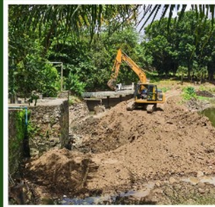
SOUTH COURSE PUMP HOUSE CONSTRUCTION GABION FILTER (ON-GOING)
