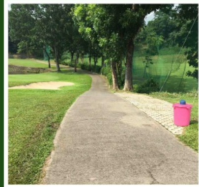
NORTH COURSE HOLE #12 CONSTRUCTION OF LAY-BY
