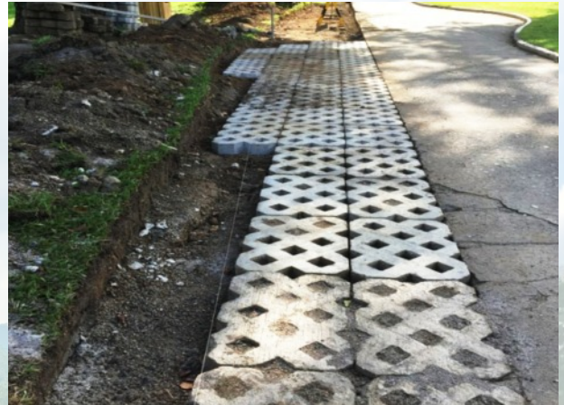
INSTALLATION OF LAYBAY EXTENSION AT TEE OFF # 13 SOUTH COURSE
