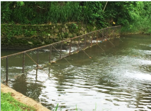
INSTALLATION OF FILTER FOR TRASH AT LAGOON # 12 SOUTH COURSE
