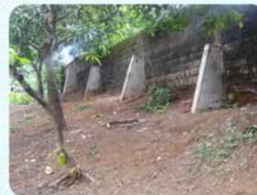
Concrete support on wall fence at Hole # 3 SC
