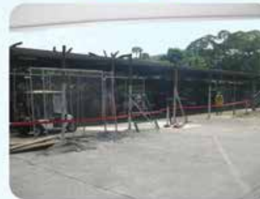
Additional Golf cart Storage before
