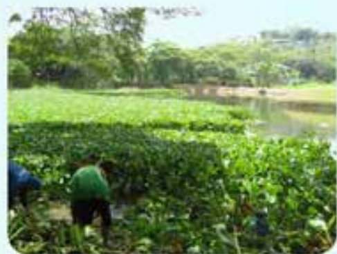
Removal of water lilies at Lagoon # 6 NC Before
