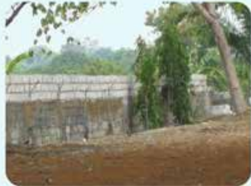
Laying of Additional chb at wall fence besides Hole # 8 SC
