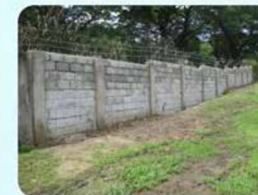
CHB fence at Hole # 3 NC After
