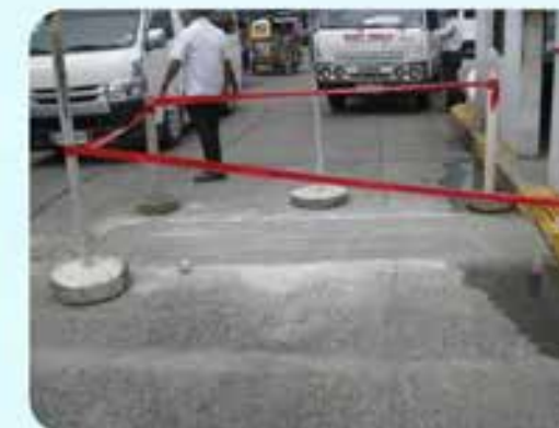
Construction of humps at Ortigas gate
